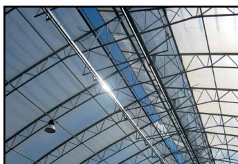
roof mounted rail
