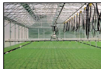
fluorescent lights mounted on the boom
